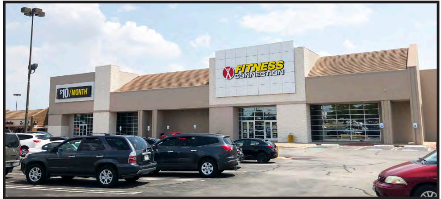
Work is underway to convert building for Fitness Connection.
